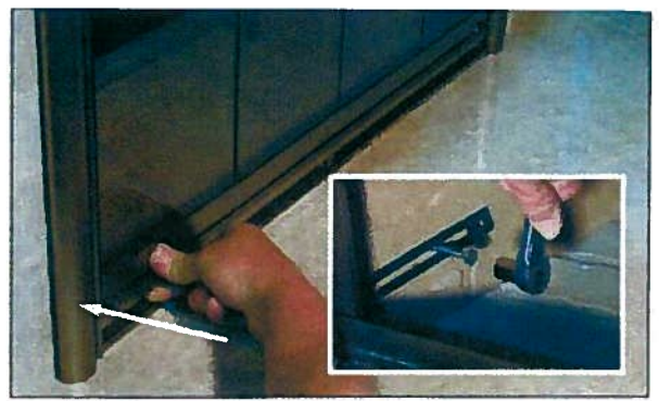
STEP 13 Move bottom of door in or out to align face of doors. Gently open doors, and tighten bottom lag bolts and lock washers. Close and recheck alignment.
