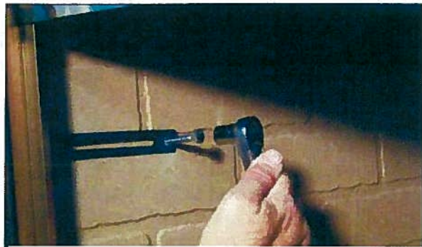
STEP 10 Install 1/4" X 1 1/2" lag bolt and lock washer into the anchor using a 7/16" wrench.
