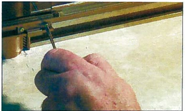
STEP 15 To adjust doors loosen set screws on back of hinge, adjust doors. Snug screws - check alignment.
